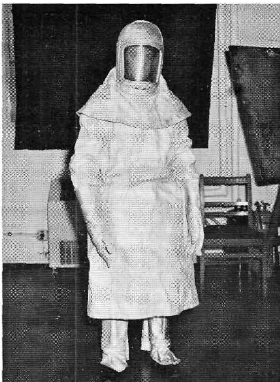
Fig. 6.—Protective clothing—aluminised asbestos
