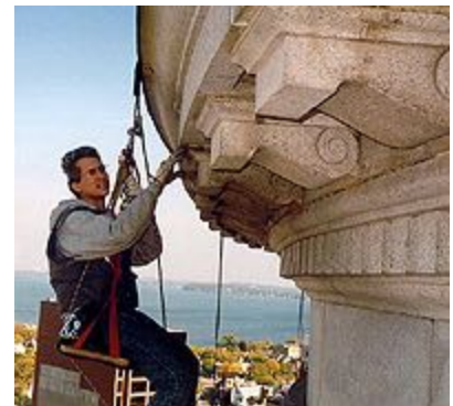
The use of special access methods may be necessary for close-up investigation of building elements. At the Wisconsin State Capitol, project architects and engineers used rappelling techniques. Photo: Wiss, Janney, Elstner Associates, Inc.
