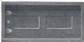
Panel in Ceiling—looking up
