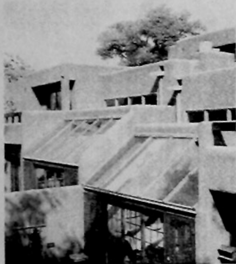
The La Vereda passive solar condominiums developed by Wayne and Susan Nichols in Santa Fe, NM., use upper-story concrete slabs and tile for thermal mass and consumer appeal.
