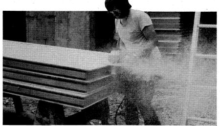
Atlas Industries of Ayer, Mass., has been making stress-skin panels for the past decade. The company has begun to market a line of low- to medium-price houses designed around its urethane foam panels wrapping laminated trusses and beams. At the building site, a workman prepares panels for splining with a router designed specifically for the job.
