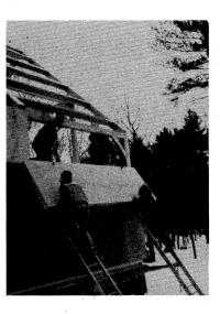
**To beef up** the thermal performance between joints, voids are filled with one-part urethane foam. The foam glues the panels together and forms an airseal. Excess is shaved off after the foam sets.
