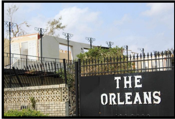
Figure 8. Loss of the roof structure with an east-facing walkway overhang. Additional lift occurred due to the overhang and to internal pressurization due to broken windows.
