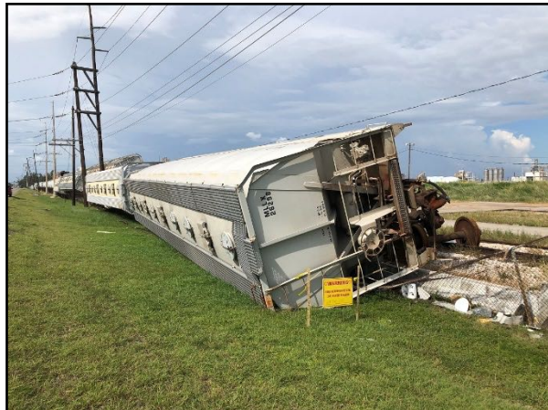
Figure 29. Overturned boxcars at the Citgo Refinery in Sulphur, LA. The cars were oriented north-south and toppled to the west with the strongest winds being from the east.
