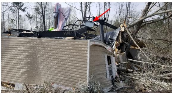
Fig. 2. Example pan system on manufactured/mobile home that experienced catastrophic failure (Overturning).
