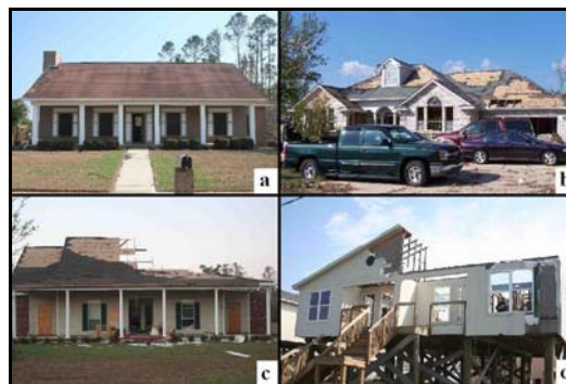
Figure 8. Various DODs to residences in Hurricane Katrina: a) loss of a small amount of the roof covering (DOD 2), b) loss of a significant amount of roof covering and some decking (DOD 4), c) removal of large sections of the roof structure (DOD 6), and removal of the roof on a residence elevated on timber pilings (also DOD 6).
