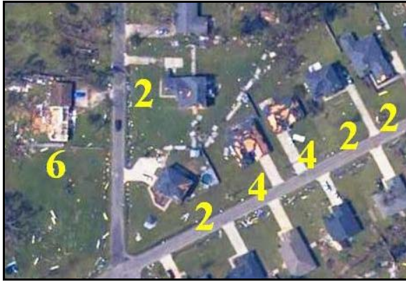
Figure 9. Various DOD numbers to residences in Long Beach, MS after Hurricane Katrina. Residences not rated did not have significant roof damage.
