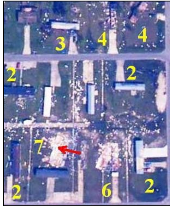
Figure 6. Various DOD numbers to single-wide manufactured homes in Long Beach, MS after Hurricane Katrina. The red arrow indicates the direction of the flipped home. Manufactured homes not rated did not have significant roof damage.
