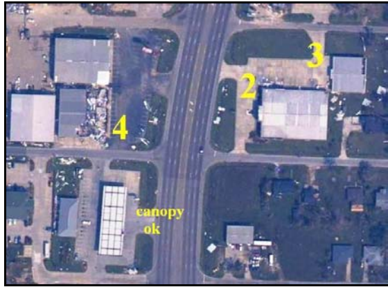
Figure 12. Various DOD numbers to metal buildings in Gulfport, MS after Hurricane Katrina. Buildings not rated did not have significant roof damage. Note the lack of damage to the adjacent gas station canopy.
