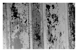
A dark layer can be seen beneath the flaking paint on these raised field panels. Depending on the project work goal and the period of the building's history being interpreted, any one of the paint layers could be duplicated in repainting. Photo: NPS files.
