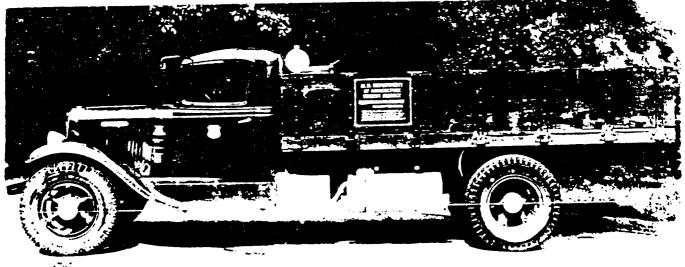
Figure 6.---Gasogen mounted on FPL truck--1942.
