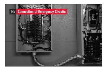
14a. Remove the main electrical distribution panel cover. Remove appropriate size knockout from the bottom or side of the main panel. (A 2-foot flexible conduit is pre-wired from the transfer switch with built-in load center). Remove threaded lock nut from conduit coupling. Feed all wires through knockout into main panel. Slip lock nut over wires and tighten securely onto conduit coupling.
