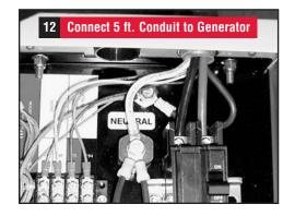
12. Access wiring connections for installation of 5 foot harness at the generator. To gain access to wiring connections and the circuit breaker you must remove the cover plate (black) above the control panel which is attached with 4 fasteners. To aid in removal it may be necessary to remove the hinge anchor bolt from the lower connection point just above the cover plate. Remove the 4 plate fasteners and remove cover plate.
