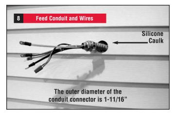
**8.** From the inside of the house, feed the end of the 30-foot conduit (INCLUDED and pre-wired from transfer switch) through the wall to outside.
