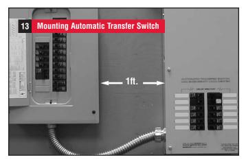
13. Locate automatic transfer switch with built-in emergency load center within one foot of main distribution panel. The automatic transfer switch can be located to the left or right of main distribution panel. Hold transfer switch against the mounting surface.
