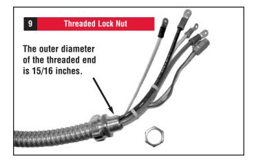
**9.** Remove the threaded lock nut from the conduit coupling.
