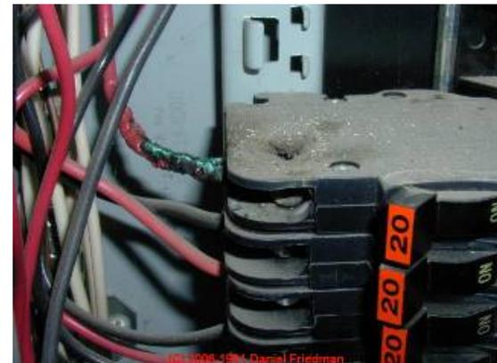
32450dsc\_0118.jpg The back side of the Federal Pacific panel cover showing melted debris where the panel touched the circuit breakers. This area was not in direct contact with the fire. The melted debris may have been caused from the failure of the circuit breakers attachment to the buss bar.
