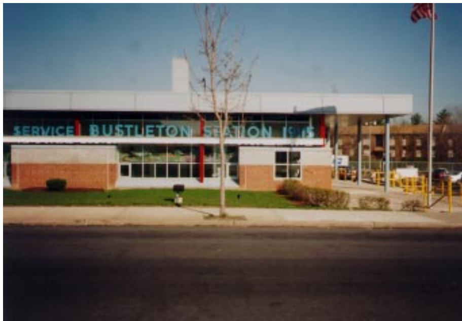
Exhibit 2 Building - West Elevation – Close Range
