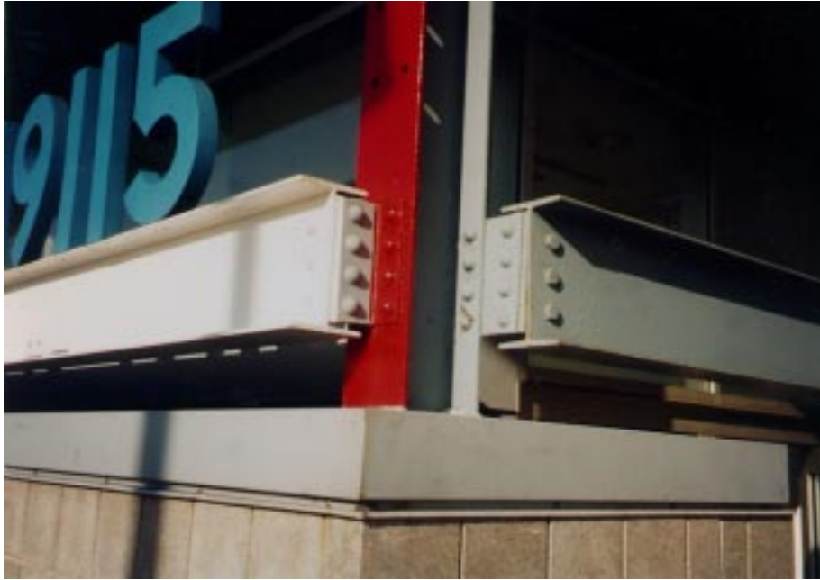
Exhibit 5 Building Construction - Detail Shot
