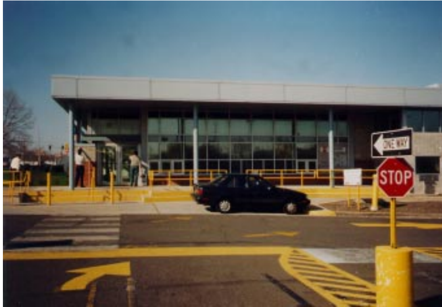
Exhibit 3 Building - South Elevation – Close Range
