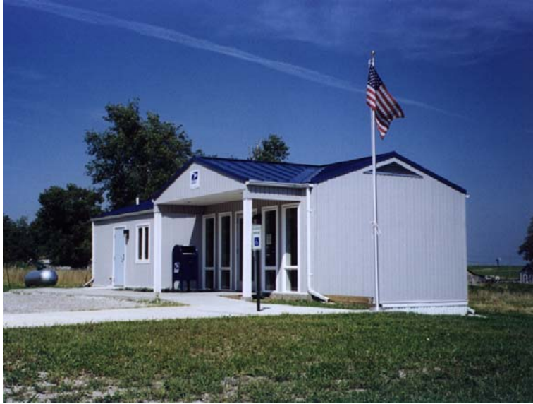
Exhibit 3a Modular Building, Eagleville, MO
