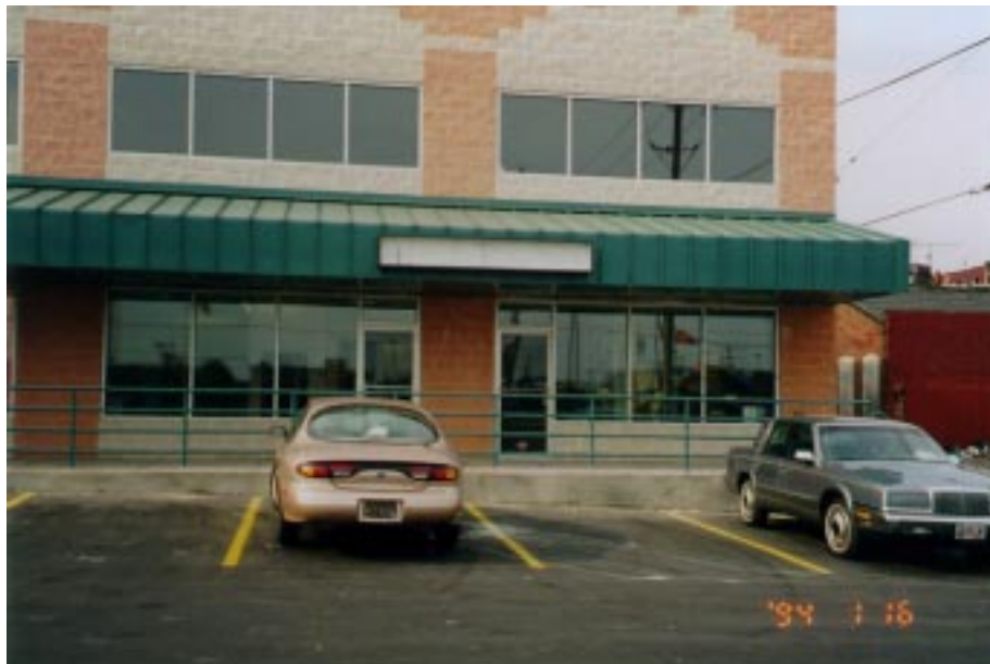
Exhibit 8 Building – South Elevation – Close Range
