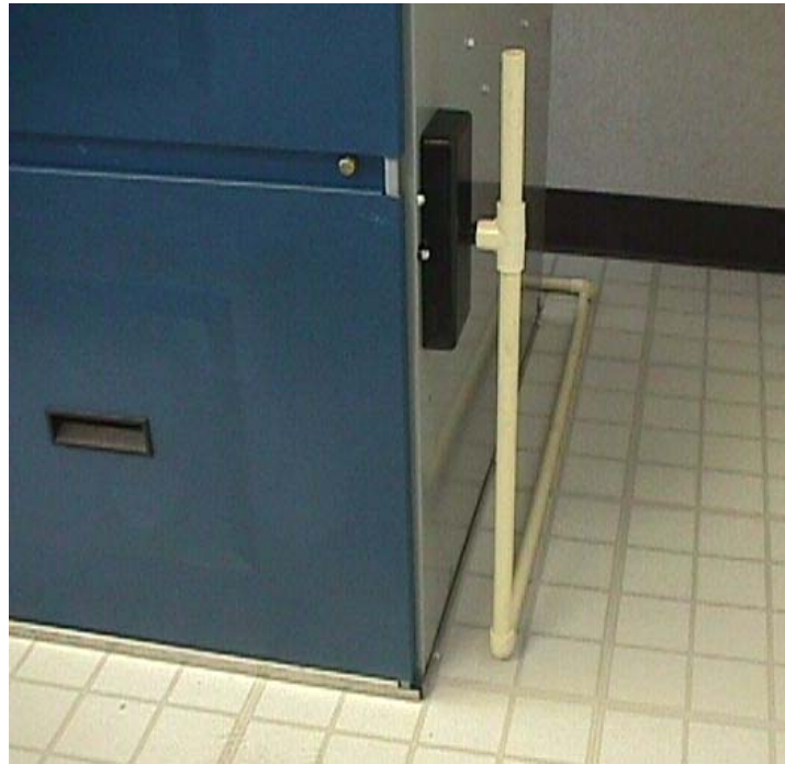
Figure 27: Condensate trap / Condensate Drainage with Vent
