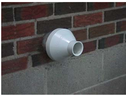
Figure 12: Concentric Venting
