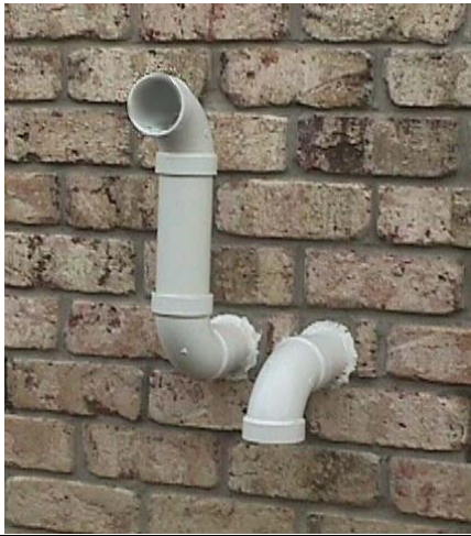
Figure 11: Periscoped Termination
