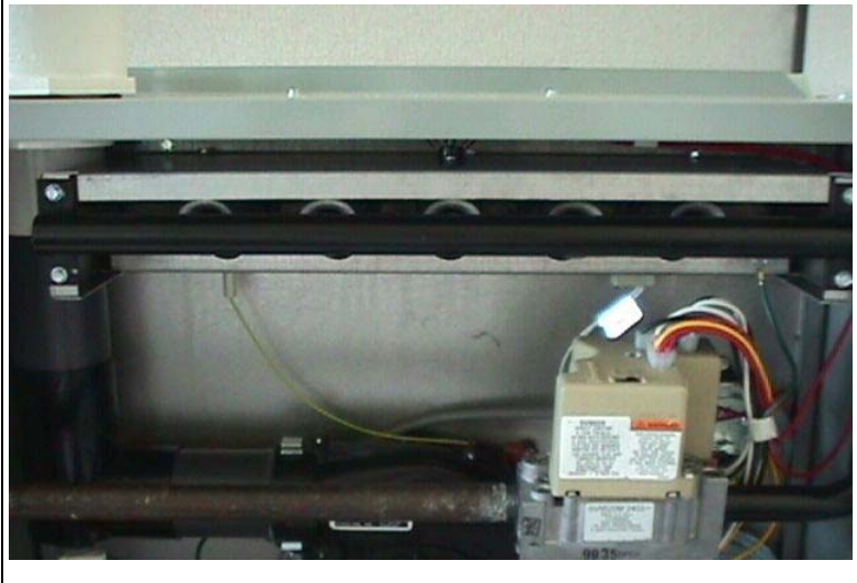
Figure 30: Inshot Burner Assembly
