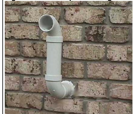
Figure 8: "Periscope" Venting
