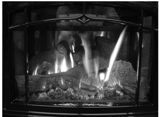
Photo 9 – Typical Burner Flame Appearance
