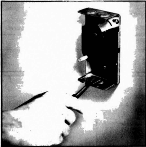
FIG. 6—REMOVING SLOTTED KNOCKOUTS.
