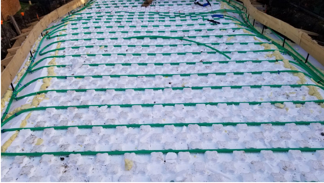
3/4in Pex Pipe for Snow Melt
