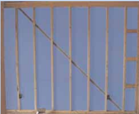
Wall sheathed with STYROFOAM™ insulation and let-in bracing.
