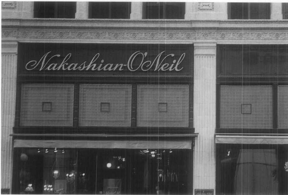
Figure 9. Panels with original tiles are shown on the left next to those featuring replacement textured glass. Photo: Chad Randl.
