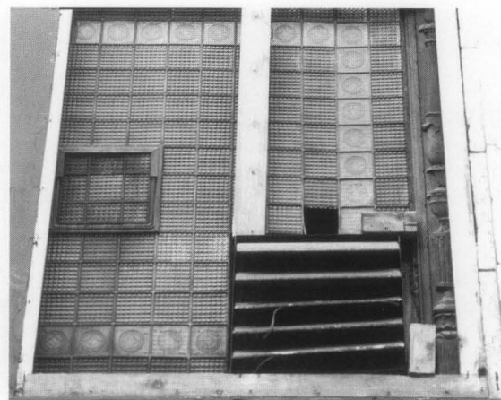
Figure 5. Transoms hidden beneath the plywood covers were in varying condition. Tiles had been removed from the panel above to fit a ventilation duct. When the panels were later rebuilt new material was needed to replace missing tiles. Photo: Oertel Architects.
