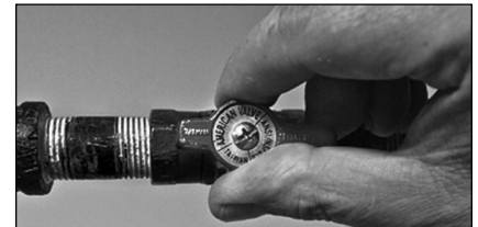
Figure 58 - Gas valve in "on" position.
