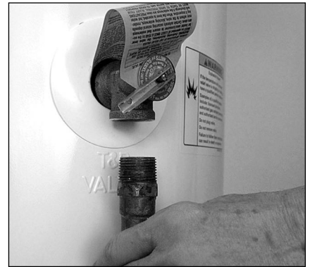
Figure 21 - Removing the T&P Relief Valve discharge pipe.
