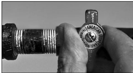
Figure 50 - Gas valve in "off" position.
