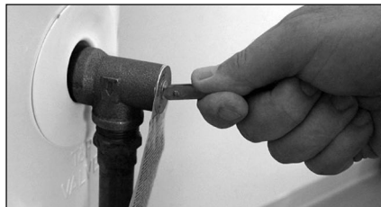
Figure 45 - T&P Relief Valve.
