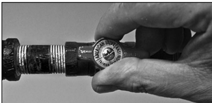
Figure 32 - Gas valve in "on" position
