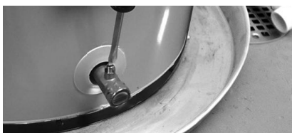
Figure 42 - Draining the water heater.
