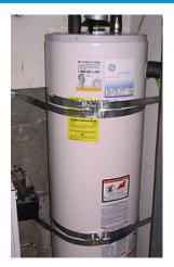
Prevent gas leaks and water damage during an earthquake by properly securing your water heater as outlined in this bulletin.
