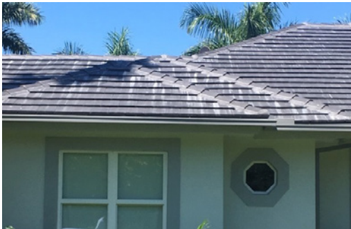
Picture of superficial efflorescence caused by the mortar installed at the ridge.
