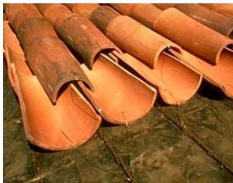
A special system consisting of brass or copper wires is used to attach these tapered barrel roof tiles. Photo: NPS files.
