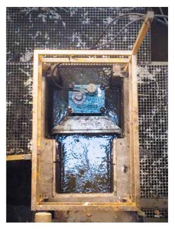
Installing new grinders at the Santa Margarita reclaimed water facility eliminated pump clogging from rag balls. JWC Environmental
