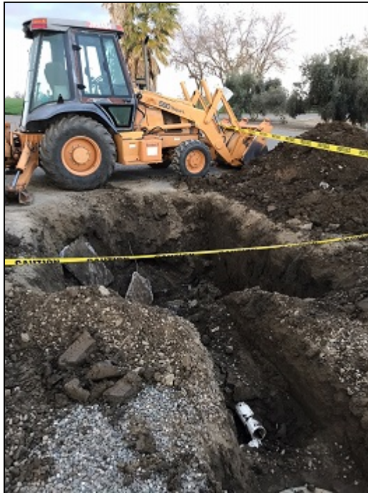
Tank backfill/burial.
