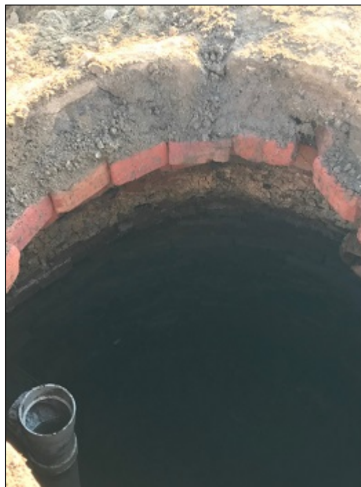
Pumped cesspool prior to abandonment.
