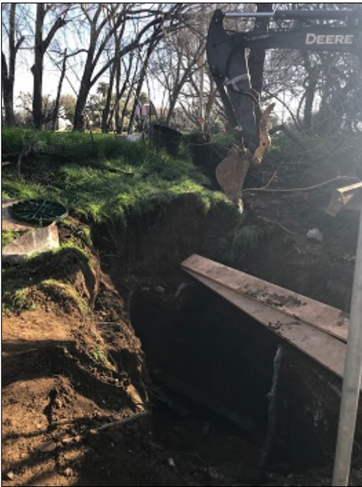
Backhoe destroying tank bottom and sides for final backfill/burial.
