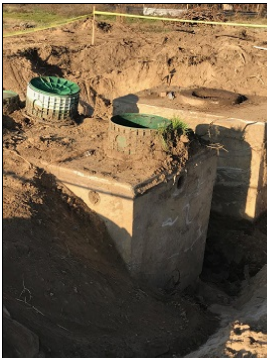
Pumped tanks available for inspection, prior to removal.
