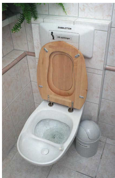
Figure 13: Urine separation toilet (BB Innovation 2002)
