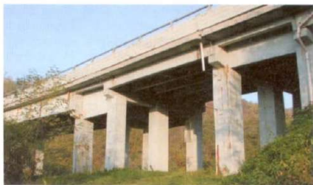
Fig. 2 : The monitored viaduct
