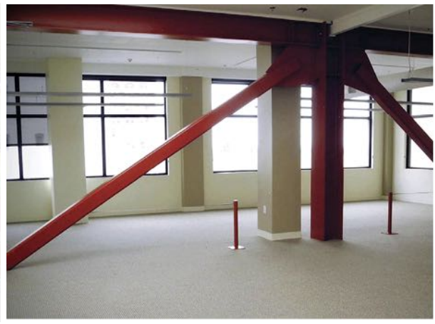
Figures 4 - 5. Using moment frames (horizontal and vertical steel members identified by the arrows) set back behind storefront openings as seen in Figure 4 (top), or placing brace frames (in red) away from the windows as illustrated in Figure 5 (bottom) are solutions that meet historic preservation goals. Figure 4. Photo: Elizabeth Hilton.
