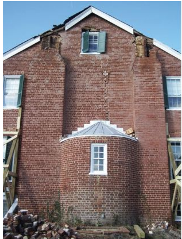
Figure 19. Chimneys are common nonstructural features susceptible to earthquake damage, even in zones of low-to medium-seismic activity as shown on this building in Virginia damaged in a 2011 earthquake. Photo: Suzanne Tripp.
