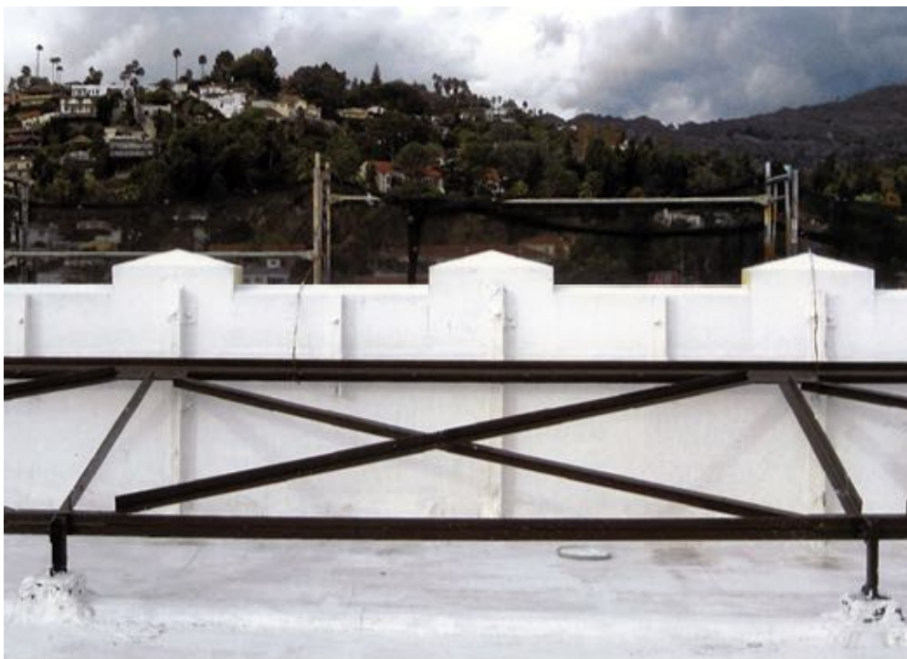
Figure 20. Bracing parapet walls, as illustrated in the typical detail drawing (top) and as installed in the image (bottom), helps avoid hazards from falling debris.
