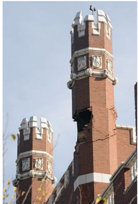
Figure 1. In 2011, a 5.6 magnitude earthquake substantially damaged all four turrets atop St. Gregory's University Benedictine Hall in Shawnee, Oklahoma. Photo: St. Gregory University.
