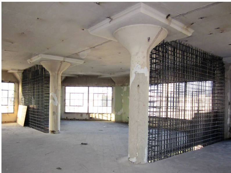
Figure 28. Steel reinforcement for the new sheer walls, perpendicular to the windows, is being installed in this concrete-frame building. Photo: Robert Chattel.
