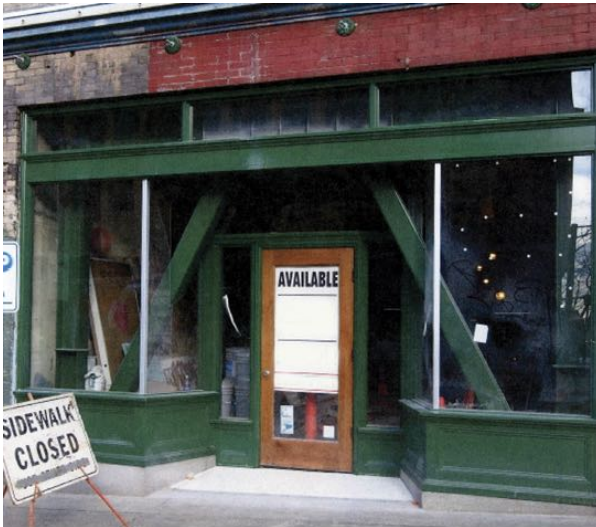
Figures 2 - 3. Standard approaches to seismic rehabilitation, such as adding diagonal bracing to reinforce window and storefront openings as seen in these photos, can be visually intrusive. Figure 2 (top). Figure 3 (bottom). Photo: Steade Craigo.
