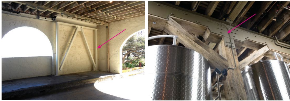
Figures 17 - 18. Careful placement of the new structural reinforcement, painted to match the surrounding building elements, if left exposed, minimizes its visual impact. New added structural elements may be left exposed when their visibility does not impair the historic character of the building. Figure 17 (top). Photo: Jason Hagin. Figure 18 (bottom). Photo: Architectural Resources Group.
