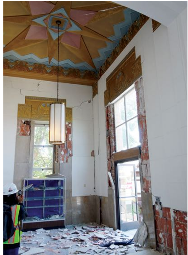
Figure 6. Failing nonstructural elements such as the stone-veneer window and door surrounds shown in this image can become a life-safety hazard when they block or impede an exit path.
