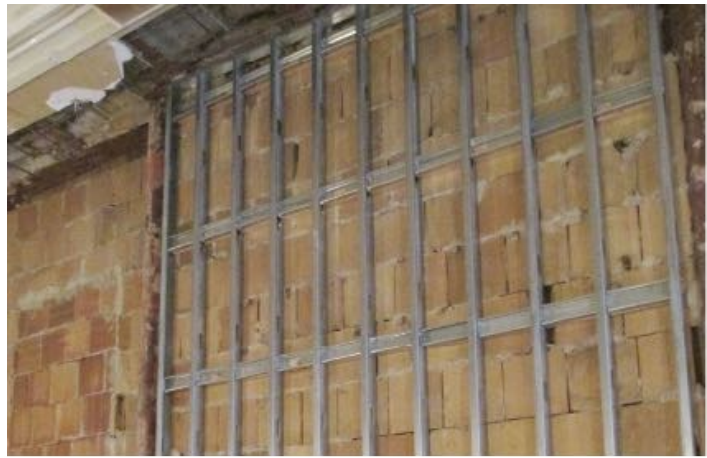
Figure 27. A new steel stud wall is being added to one side of this interior hollow-clay tile wall. The side with the least amount of historic finishes was chosen as the least disruptive location for the added reinforcement. The wall will be returned to its original appearance by installing new finishes matching the historic finishes. Photo: Wiss, Janney, Elstner and Associates, Inc.
