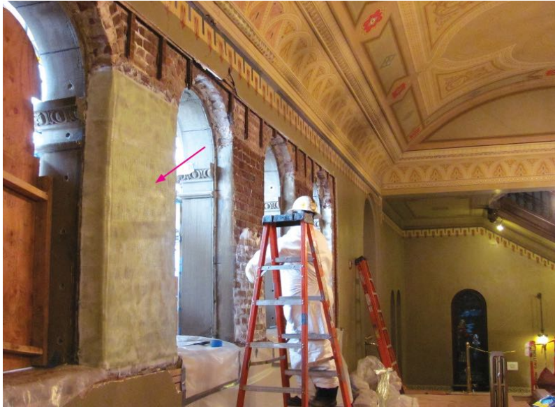
Figure 26. Epoxy-embedded fiberglass mesh is being bonded to the back of the brick pilasters of this 1906 unreinforced masonry building. New finishes matching the appearance and detailing of the original finishes will be applied over the mesh.
