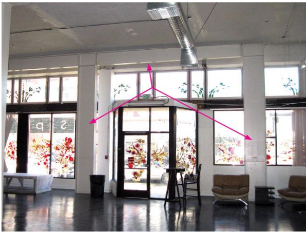
Figures 4 - 5. Using moment frames (horizontal and vertical steel members identified by the arrows) set back behind storefront openings as seen in Figure 4 (top), or placing brace frames (in red) away from the windows as illustrated in Figure 5 (bottom) are solutions that meet historic preservation goals. Figure 4. Photo: Elizabeth Hilton.
