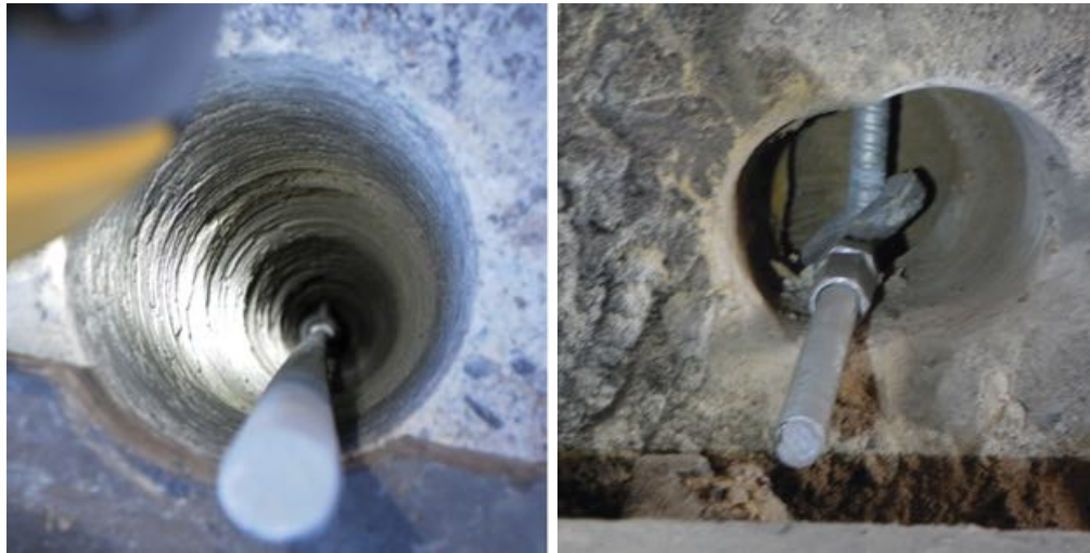
Figures 23 - 24. View of one of the center cores drilled down through the wall (top). Eye bolts are used to anchor the floor to the wall (bottom).
