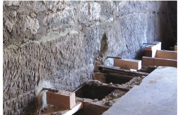
Figure 25. Location of the eye bolts after grouting. The seismic rehabilitation of this historic wine cellar building shown in Figure 21 included center coring of the exterior stone walls to add steel reinforcement, as illustrated in Figures 22 and 23. The floors were tied to the steel reinforcement in the walls using eye bolts, as seen in Figures 24 and 25, eliminating the need for exterior washers or plates. Figure 21. Photo: Architectural Resources Group. Photos: MKM & Associates.
