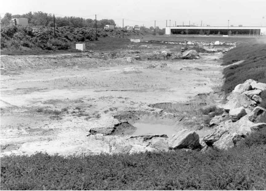
Figure 16. Sinkholes in a storm-water retention basin along U.S. Route 22 in Lehigh County.
