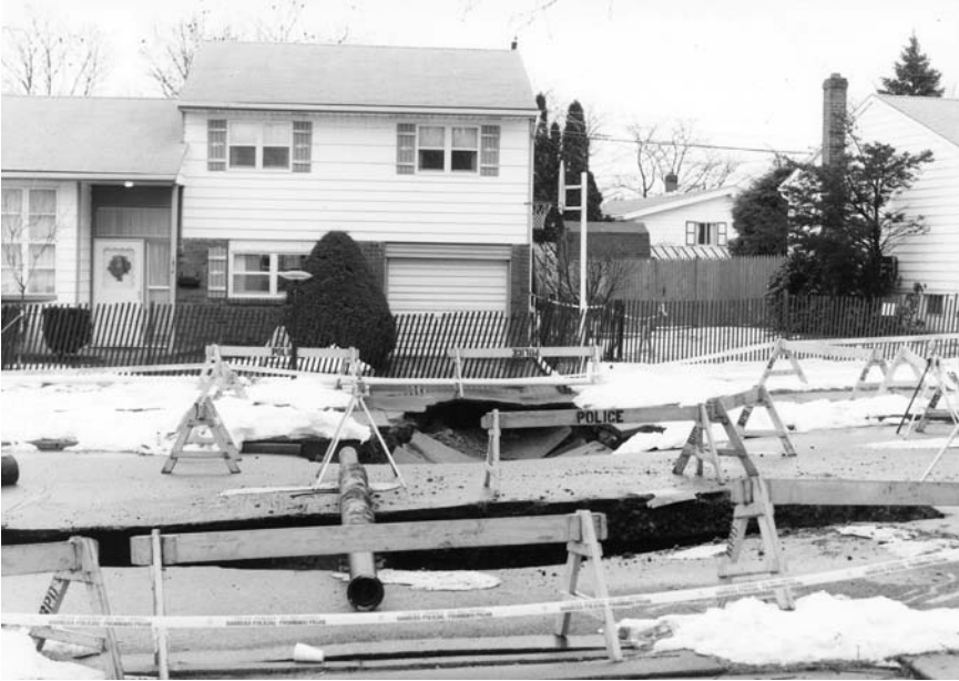
Figure 17. Sudden collapse of a city street attributed to a water-line break in the karst area of Northampton County.
