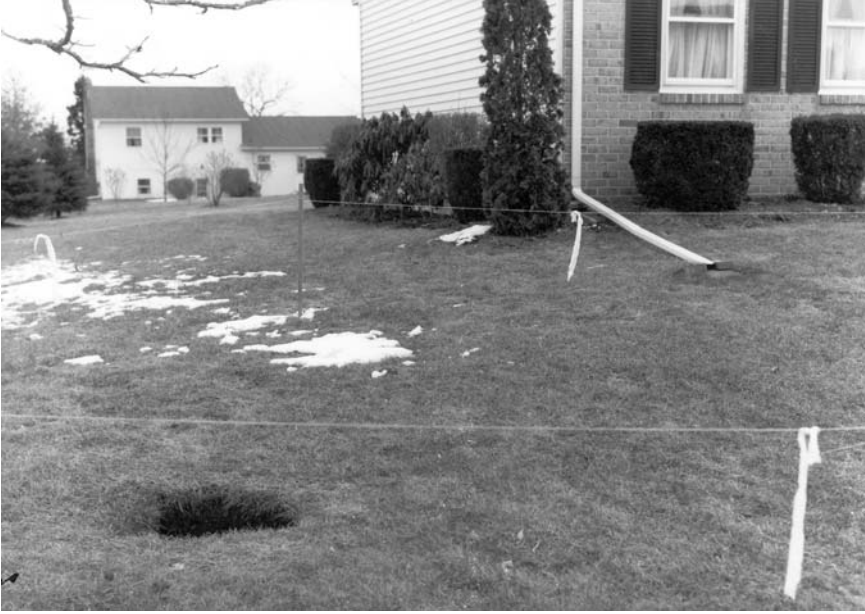
Figure 15. A sinkhole resulting from water discharging from a storm gutter. Sinkhole formation can be attributed to storm-water runoff throughout central and eastern Pennsylvania.
