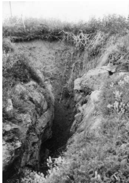
Figure 11. A sinkhole having an open drain.
