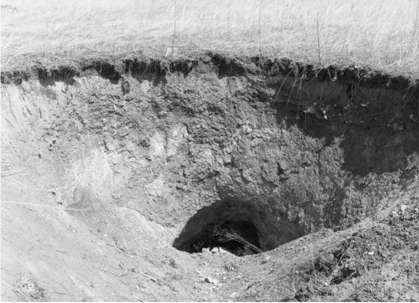
Figure 10. A shallow sinkhole showing the throat and soil arch.
