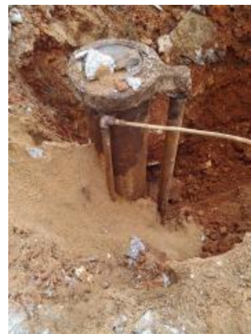
Domestic water wells typically have steel or PVC casing.
