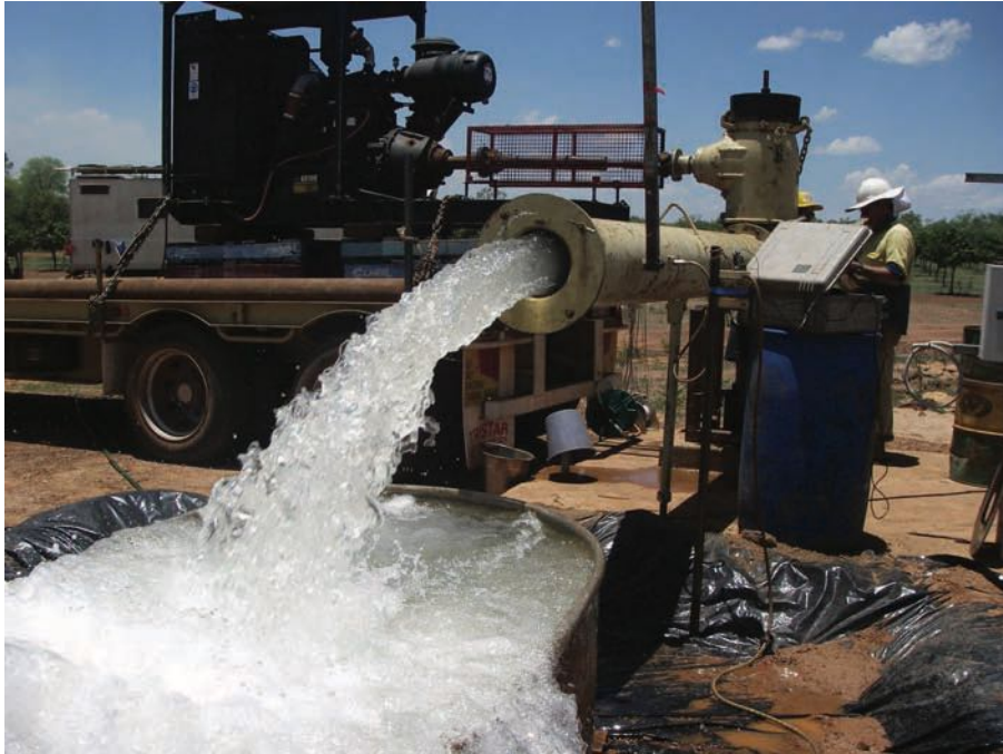
Test pumping an irrigation bore
