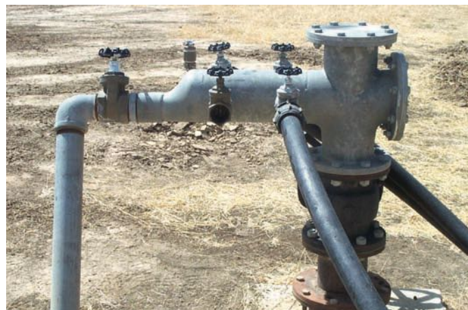
Water supply under control
