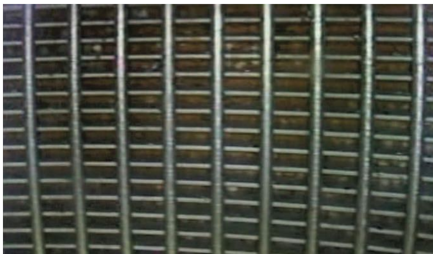
Downhole images of screens and gravel packs published with permission from Age Developments Pty Ltd
