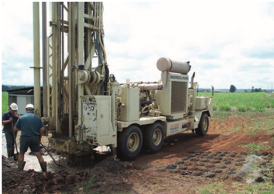
Laying out samples of drill cuttings
