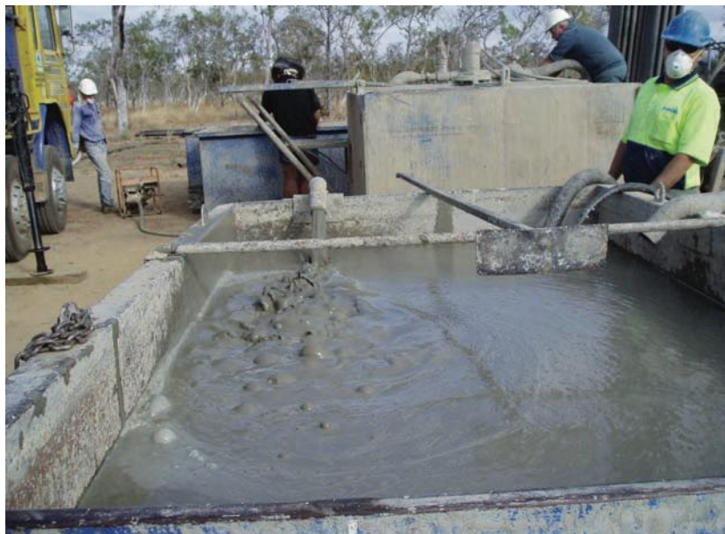
Cementing the bore
