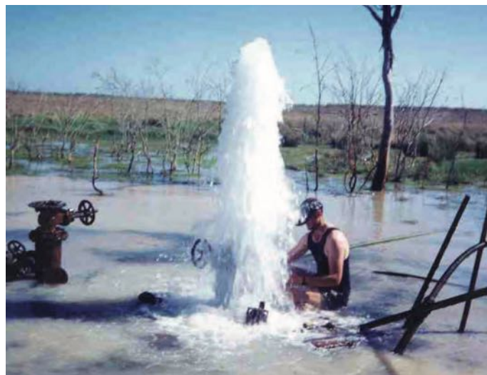
Water supply out of control
