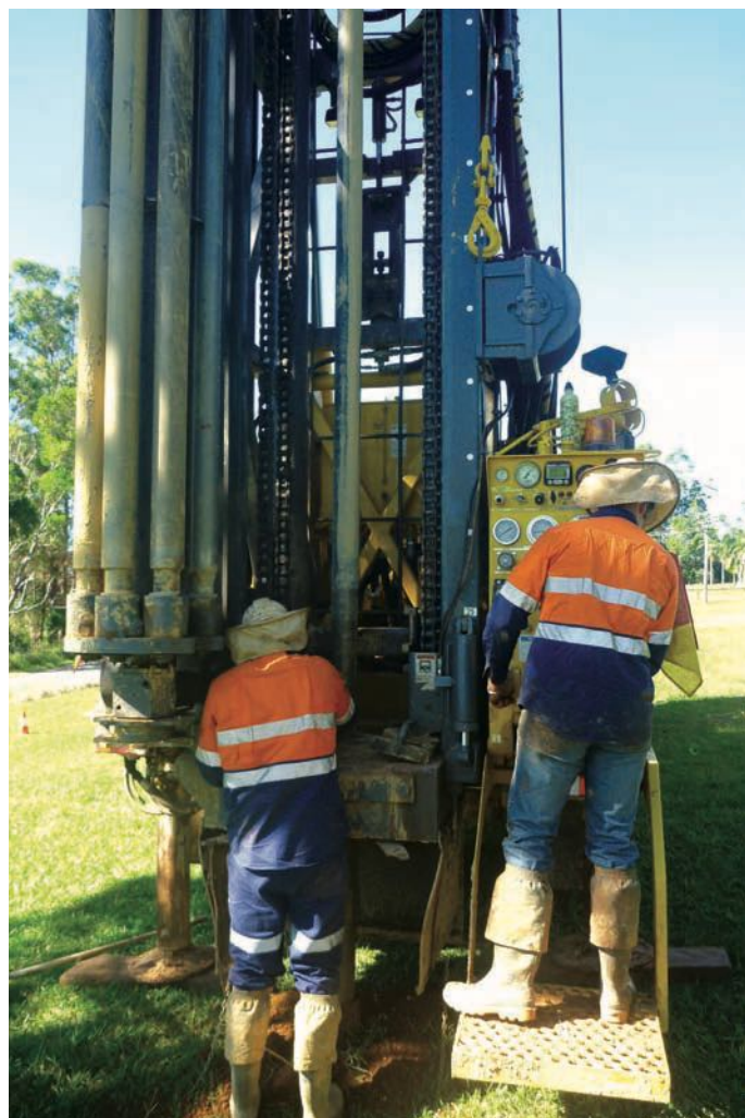
Rotary air drilling
