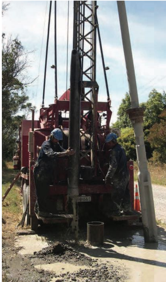
Cable tool drilling
