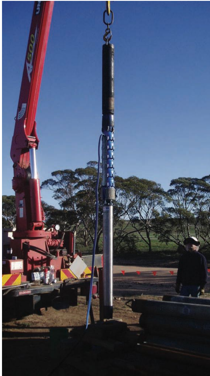
Submersible pump being lowered into a bore
