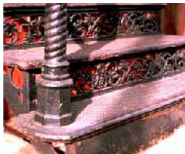
The risers on these cast iron steps feature a highly decorative pattern. Photo: NPS files.
