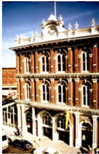
The west facade of the New Market Theater retains its original cast iron features. Photo: George McMath.
