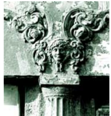
Cast iron feature in need of cleaning and painting. Photo: Courtesy, New York Landmarks Conservancy.
