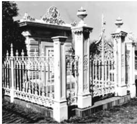
The Slatter Family Tomb in Mobile, Alabama, consisting of a cast-iron mausoleum and fence, exhibits the wide range of uses of the material in the 19th century. Photo: Jack E. Boucher, HABS Collection.
