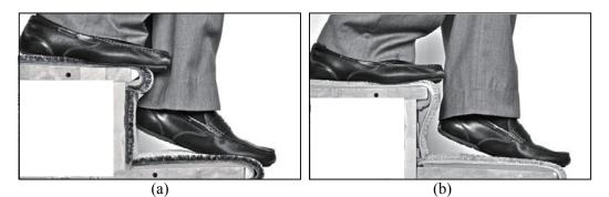
Figure 2. Mockups of (a) typical Canadian home stair and (b) typical public stair, both carpeted but with different carpet treatments that would meet typical code requirements prohibiting abrupt lips of projecting nosings, but only on public stairs
