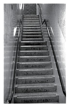
Figure 4. Hundreds of marks on stair risers due to heel scuffs, some of which occurred during descent in a high-flow evacuation drill in 1971.
