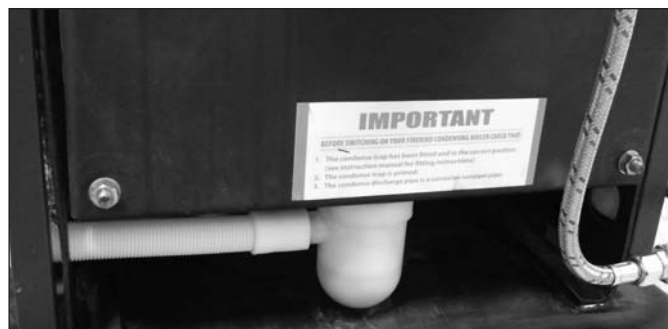
The condensate trap is located at the base of the boiler
