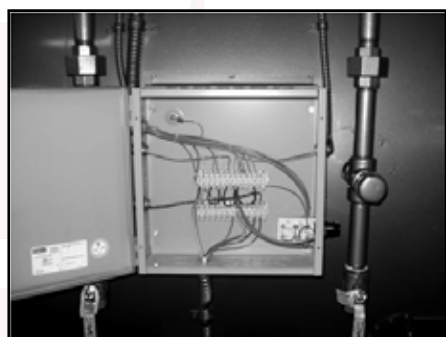
Example 12" x 12" junction box With terminal strips Figure 39a
