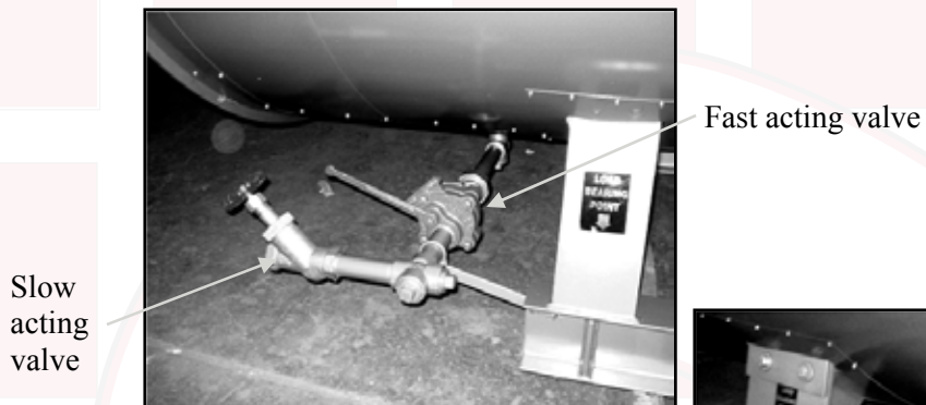
Blowdown valves, single connection: Figure 33
