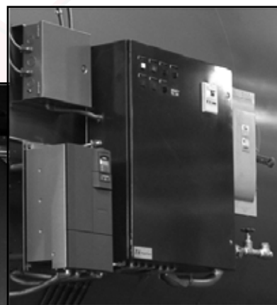
Example of multiple junction box's including: Burner control panel, power disconnect, VFD controller, and junction box, Figure 39c
