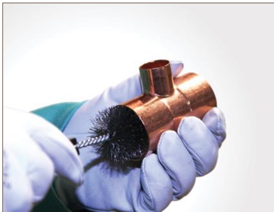
Figure 7.8. Cleaning: Fitting Brush
