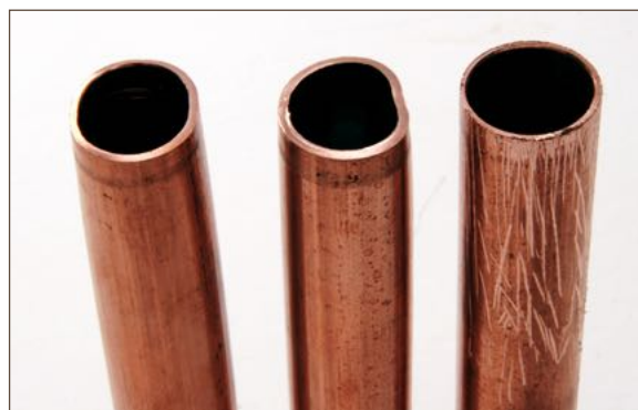
Figure 10.1. Inspect tube for imperfections
