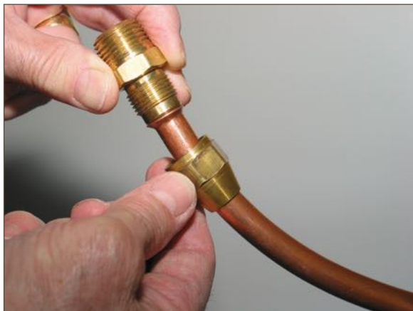
Figure 9.1. Flare Fitting/Flared Joint During Assembly
