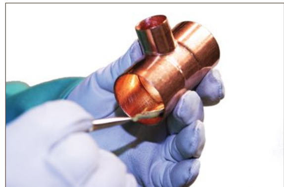
Figure 7.10. Fluxing: Fitting
