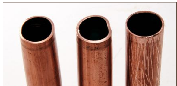
Figure 11.4. Inspect tube for imperfections
