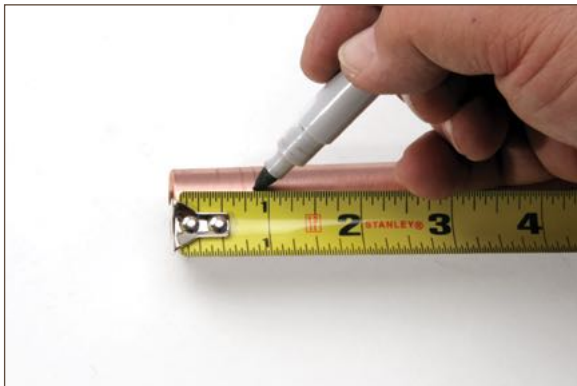
Figure 11.12. Measuring depth of insertion
