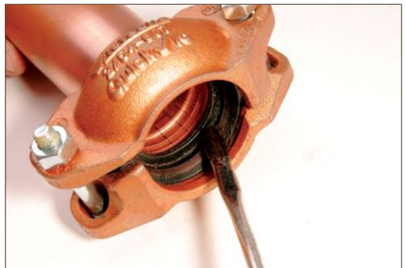
Figure 10.8. Applying lubrication to gasket
