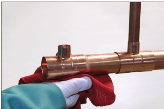
Figure 7.12. Removing Excess Flux
