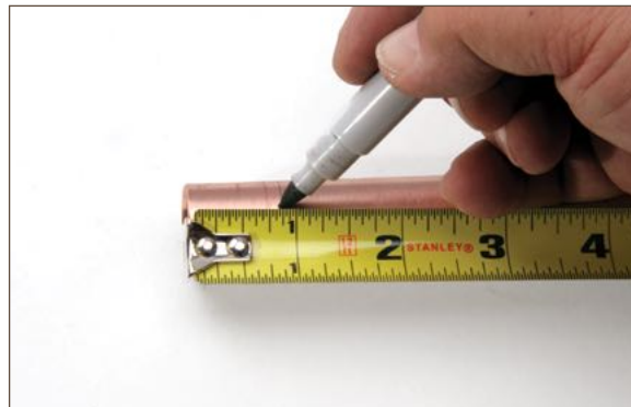
Figure 12.10. Making insertion depth
