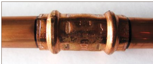
Figure 11.16. Completed installation of a press-connect joint
