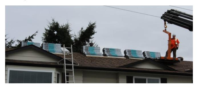
In the image above, you can see that the roofing team is unloading the shingle bundles with the help of a conveyor. The shingle bundles have been stacked correctly. If you were to stack the bundles higher than shown here, therefore concentrating the load of many bundles in a small area, you may cause long-term issues with the roof structure.
