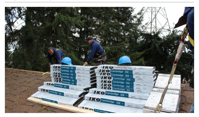
Some contractors will intentionally stack the shingle bundles over the roof's ridge. They may call this process "breaking the bundles," which may help separate <u>3-tab shingles</u> from one another. However, you must do this carefully. If you drop the bundles with force, you may damage them or the roof, especially in cold weather.
