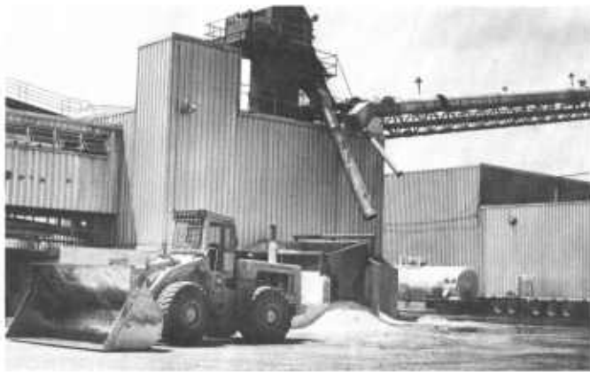
Figure 68—Facility for feeding stored chips into conveyor system, bypassing the woodroom.
