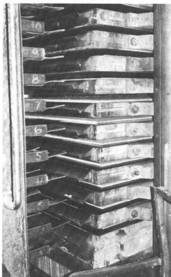
Figure 185 —Loading of S2S press. Mats in position are about 1/2 in thick. Press ready to close.
