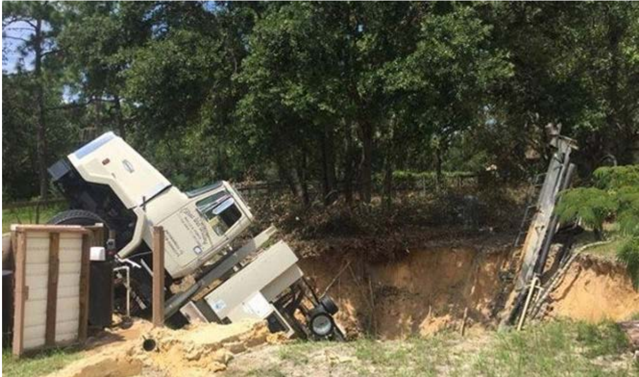
Figure 6. A sinkhole triggered during well drilling damages rig. (photograph credit Bay News 9, Tampa)
